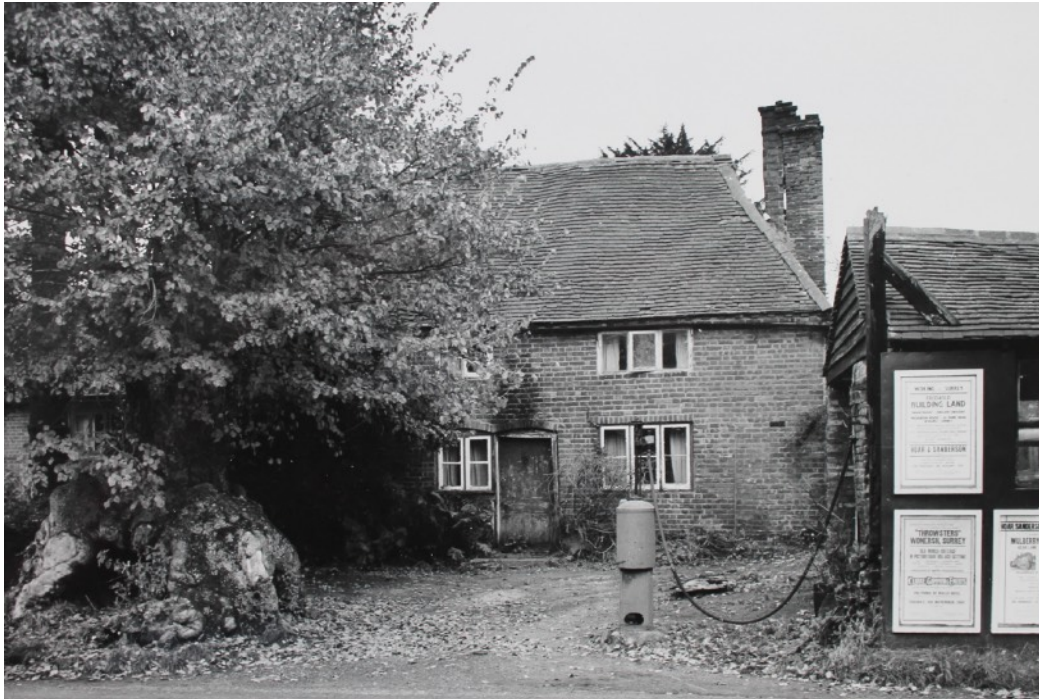
The Old Forge in 1969 showing the chimney that was built in the late sixteenth century when the open hall was divided.
